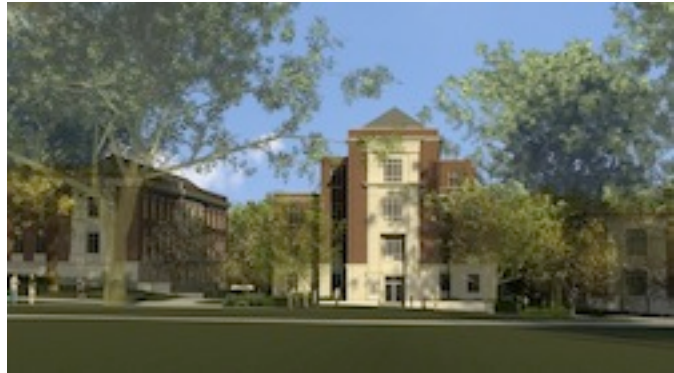
Figure 1.2.1: Old Main Mall Entrance
